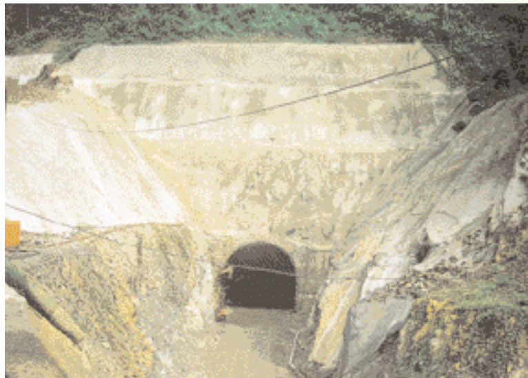
The Da Mi site: Nearing completion, it will be operational in 2001.
