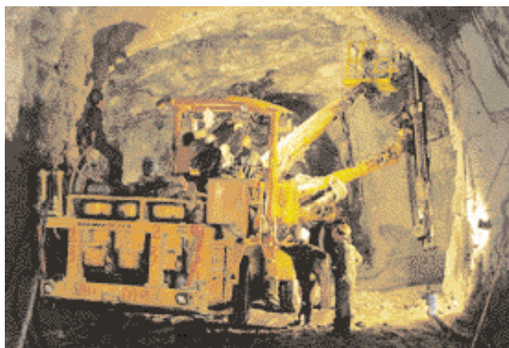
At the Hâm Thuãn site: An Atlas Copco Boomer H175 drill rig, one of four similar units handling the drilling there.
